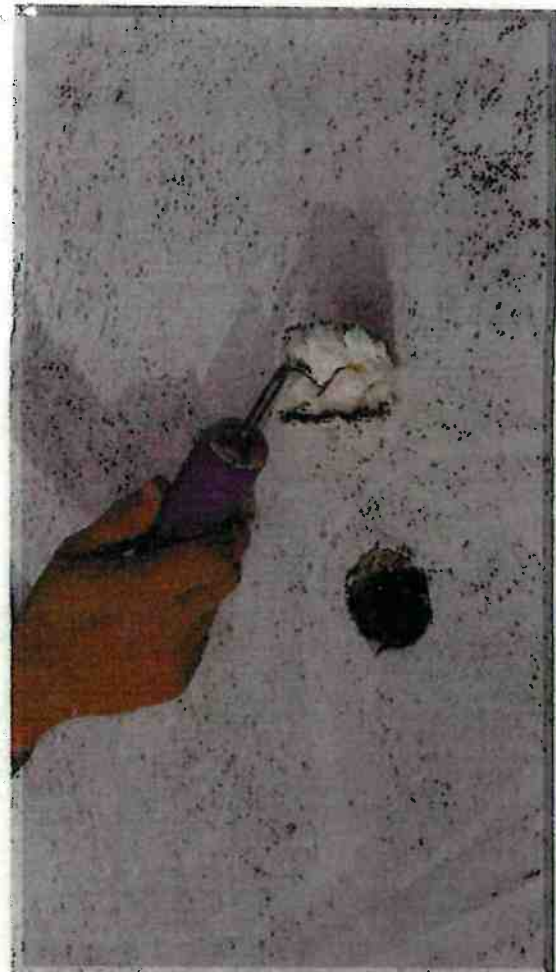
Photo 75 - 2" core showing membrane & insulation
